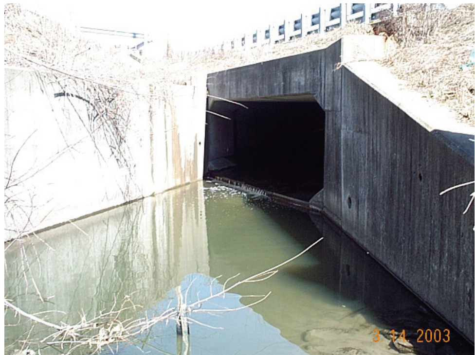
Figure P.3.17 Culvert Skewed End
