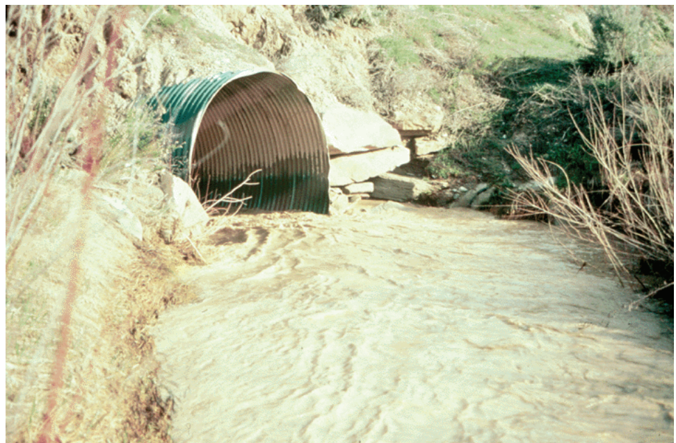
Figure P.3.15 Culvert End Projection
