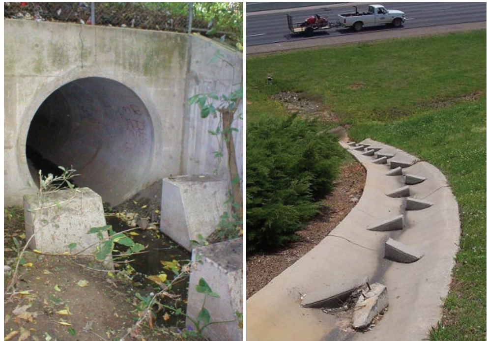
Figure P.3.20 Energy Dissipator
