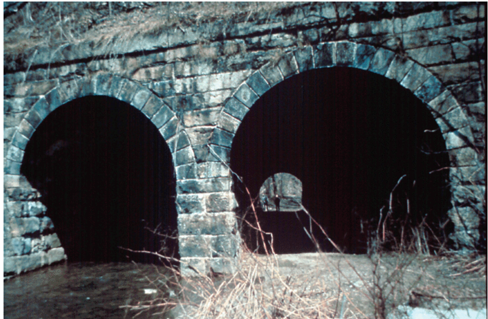
Figure P.3.13 Typical Stone Masonry Arch Culvert
