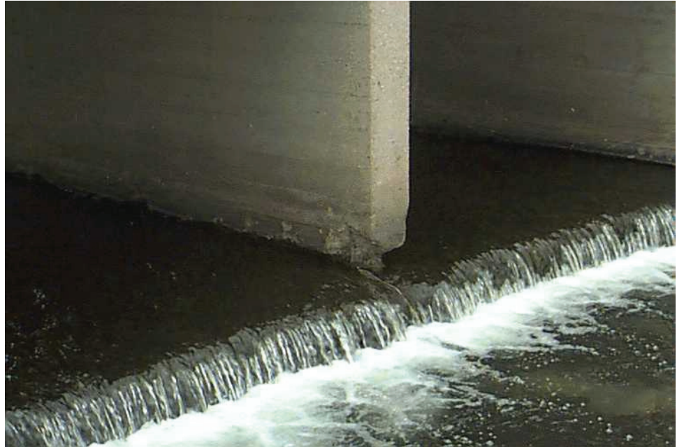
Figure P.3.34 Energy Dissipater
