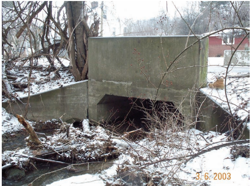
Figure P.3.32 Culvert Headwall
